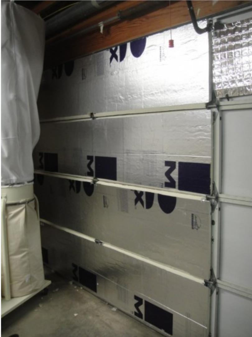
Here's where I did a mock-up to see if each panel fit; each one is custom cut because I found variations in the dimensions. Note the chamfer between panels to allow the door panels to pivot when it opens along the track.
