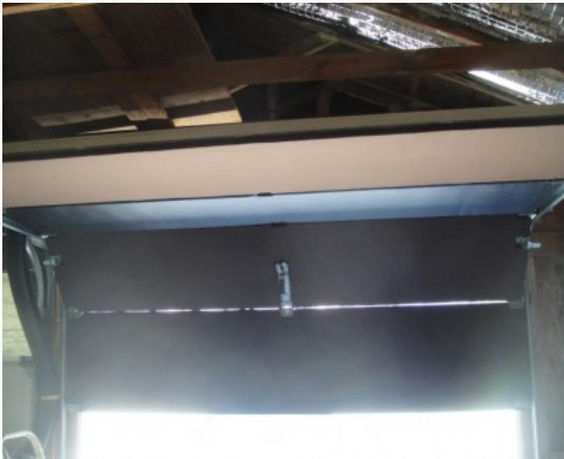
I added a strip of foam adhesive tape to the seams between the door panels to keep the door sealed when closed. The rubber seal around the door edges is kept tight by adjusting the track closer to the door frame but still allowing it to slide.
