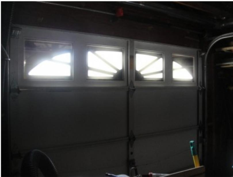
The windows add to the heat in the shop; before I made the panels I had a section of radiant barrier taped over the windows with gaffer's tape.
