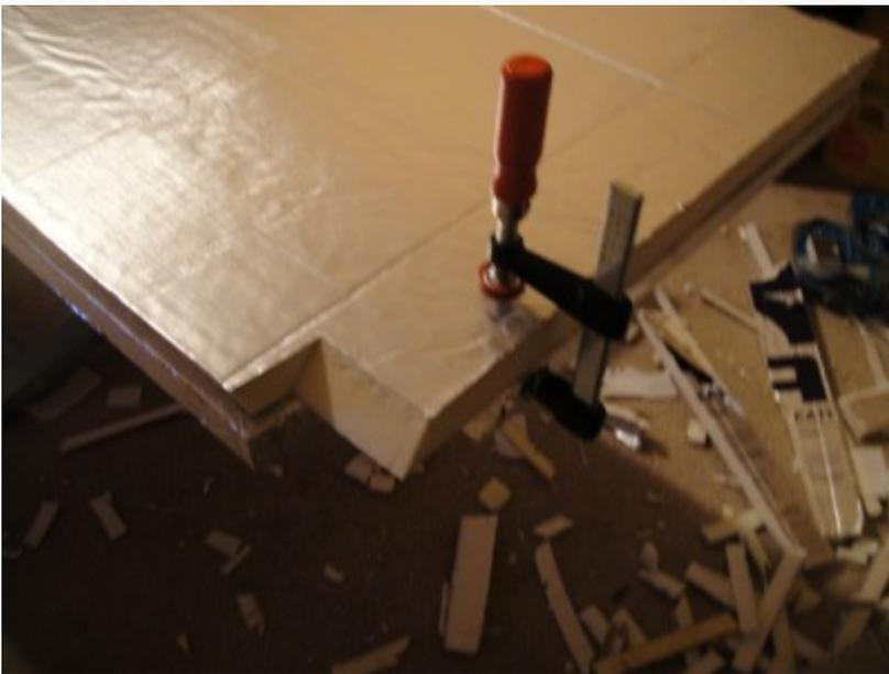
What took some time is custom-cutting around the hinges. Kind of a trial and error thing, like sneaking up on miter cuts.
