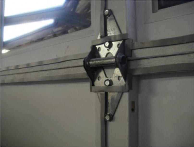
I used weather seal tape to add a cushion to the panels, and to help keep the sunlight from leaking through. While you may not get a complete air seal from the panels, you can get pretty close.
