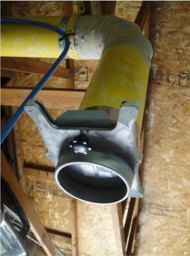
Each tool will get a blastgate. This one I've sealed the edges to help keep leaks to a minimum.
