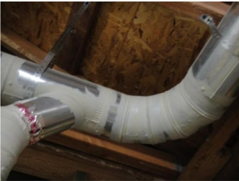
By using long-radius elbows, you give the air a gentle sweep to travel in, reducing static pressure (resistance to airflow), and you get more airflow (CFM) out of it.
